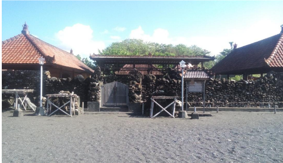
Figure 1. Hyang Sangkur Temple front view located in the Subak Biyaung area of Gianyar Source: Document I Nyoman Sama, dated 10 May 2016
