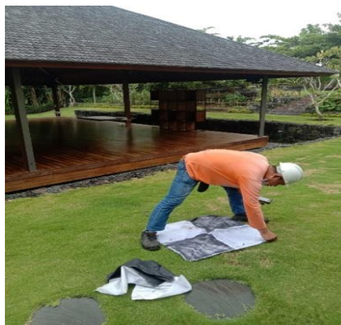
Figure 4. Setting up premarks for ground control point measurements
