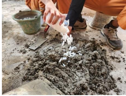
Figure 4. Paving block sample generation
