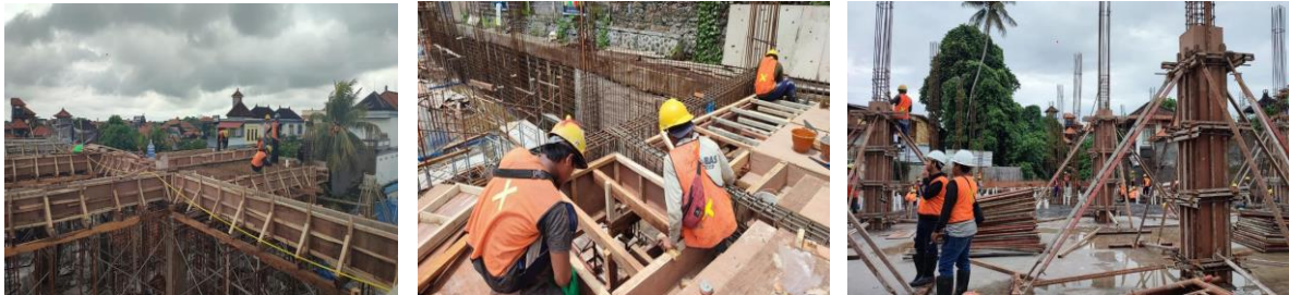
Figure 3. Formwork installation
