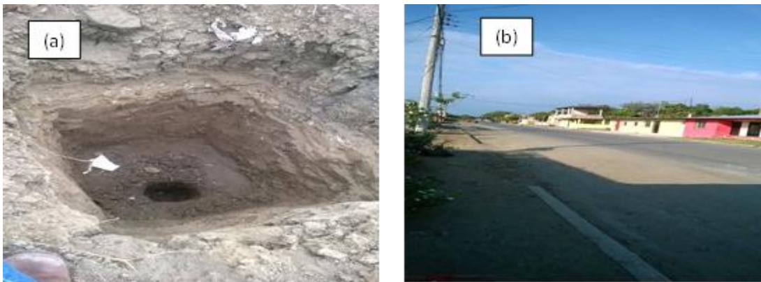
Figure 1. Open pit test of 1m 2 (a) at Eloy Alfaro Street (b)
