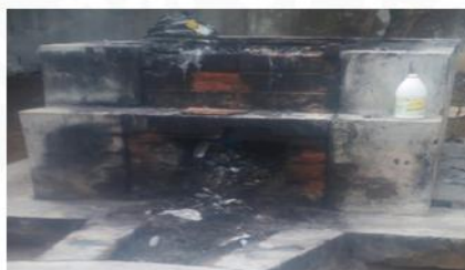
Picture 3. Incinerators used for destroying biomedical waste
